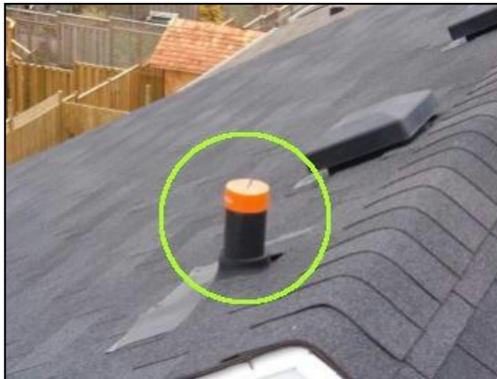
Plumbing stack is capped
