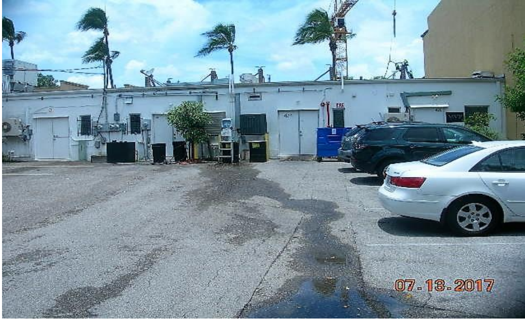
Rear View – 14-parking spaces
