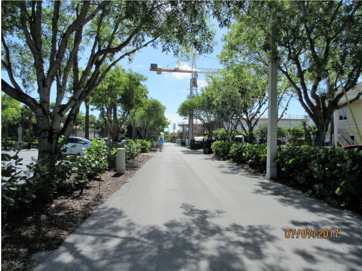
Service Alley 20' ROW – Subject on Left side of this photo
