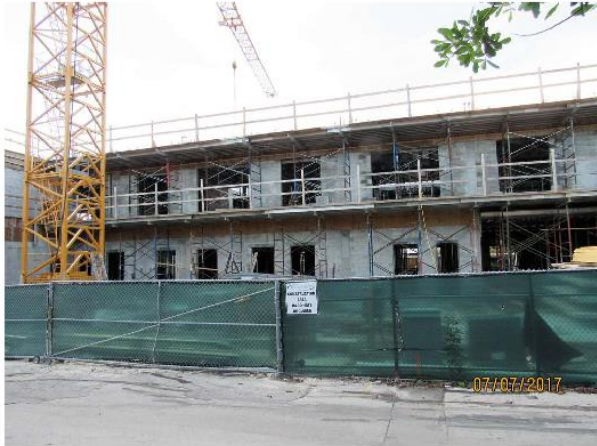
5th. on 5th. under construction - south of alley
